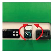
Toggle the boiler switch to turn it ON and OFF.
